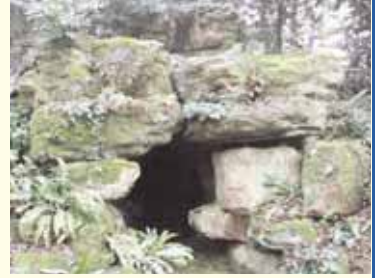
Artificial stone (Pulhamite) cave of the mid C19th designed specially for Highnam Ct Grade II
