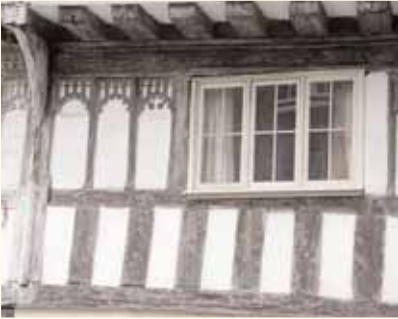
Detail of cusped arches, 82/83 Church St, Tewkesbury, Grade II*
