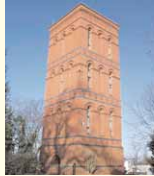
Mythe Water Tower, Grade II, built 1889
